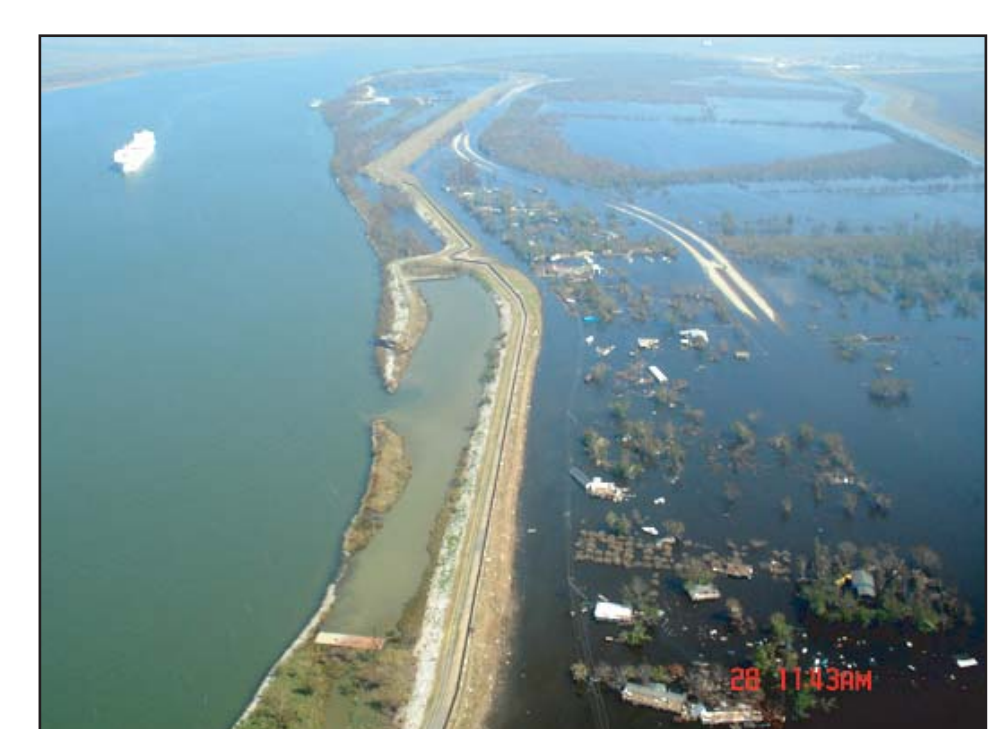
Mississippi River near Boothville, Louisiana, showing damage resulting from Hurricanes Katrina and Rita.
