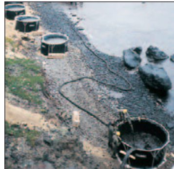
Oil wastes in temporary storage near a shoreline.
