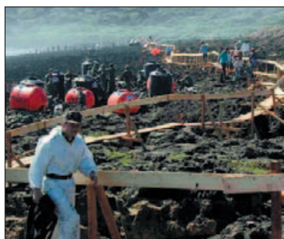
Providing safe access to the worksite is critical to reducing the risk of accidents.
