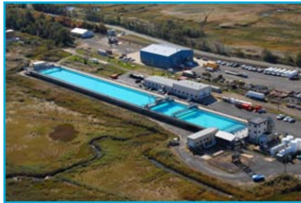
Figure 1. OHMSETT test facility.
