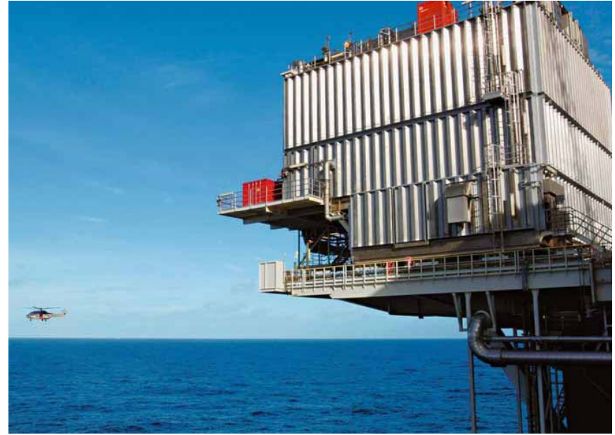
HVDC Light Module on Troll-A platform (ABB)
