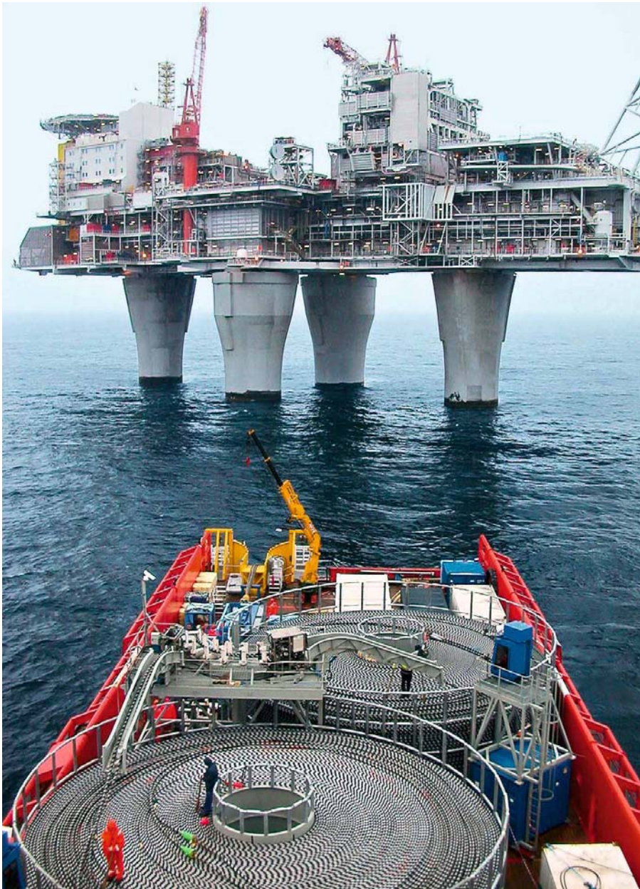
Troll-A oil platform in the North Sea and cable laying ship (ABB)
