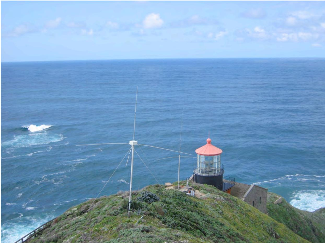
Figure 1. View of the receive (foreground) and transmit (background) antenna elements for the SeaSonde™ HF radar system deployed above the lighthouse at Pt Sur, California. The system and communication electronics are deployed in a small, weatherproof enclosure below the transmit antenna.
